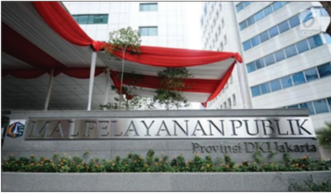
Fig. 1: MPP mall view Source: Doc Pemda DKI
